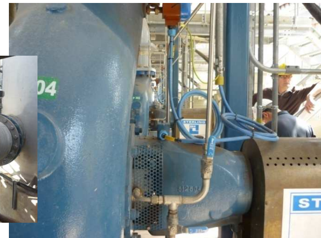
Transnorm centrifugal pumps (7 off)
